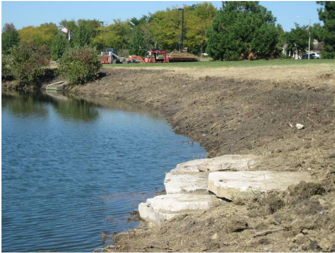
Stone pond access platform installed
