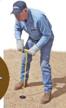
Pull up on the hook, rotating the anchor to the locked position.
