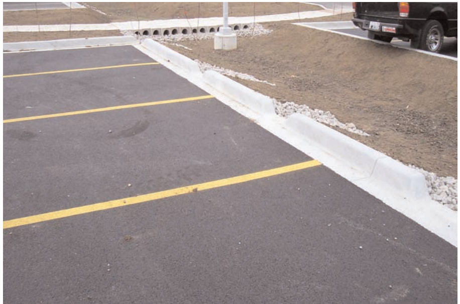
Landscaping being installed in, and along the drainage swales.
