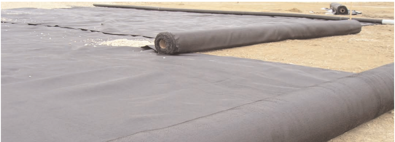
Mirafi® HP570 being rolled out with an 18” overlap.
