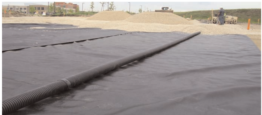
Drainage pipes laid during aggregate placement.
