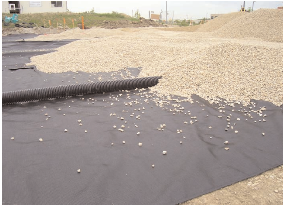
Open graded stone being placed over the drain tiles.
