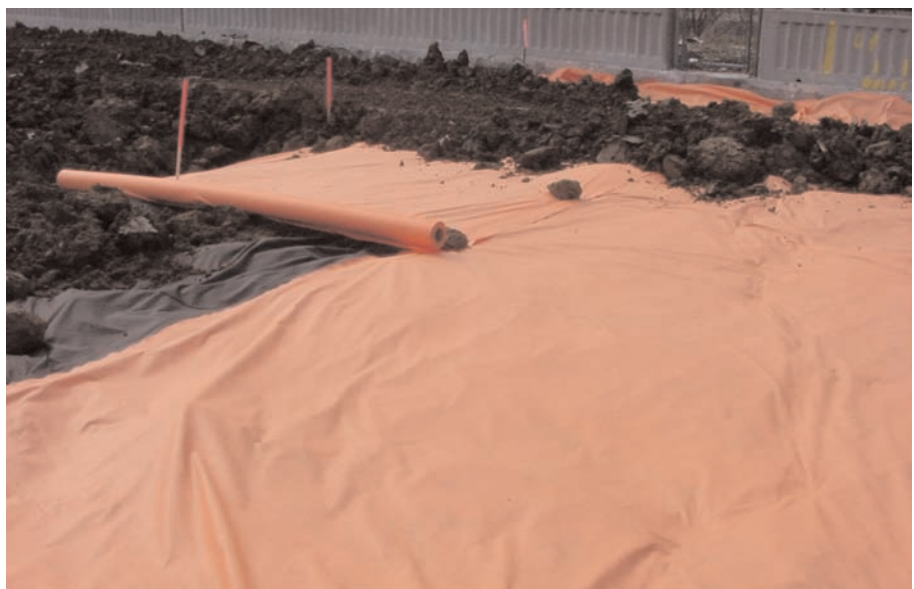
Placing Mirafi® Orange delineation fabric.
