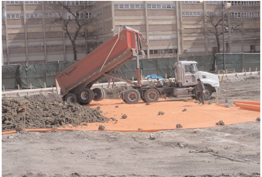
Subsoil condition prior to installation of Mirafi® MPV500.
